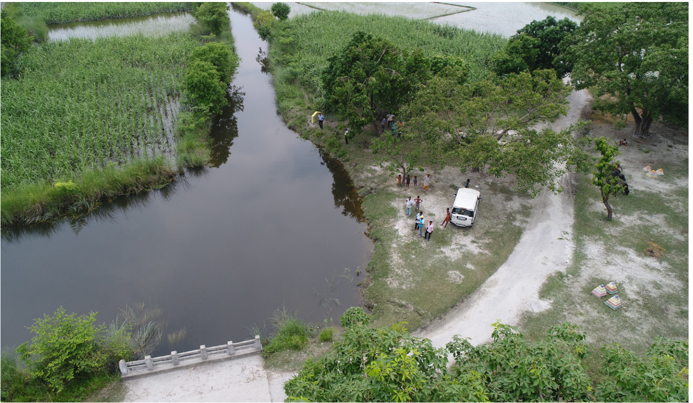
A renovated water channel (called 'pyne'), supplying irrigation water to agricultural fields in a peri-urban locality
