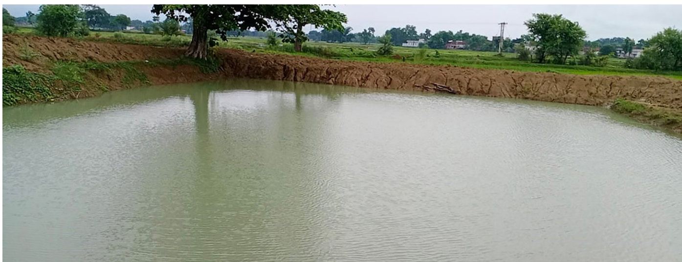
Pond constructed in a peri-urban locality to conserve rainwater
