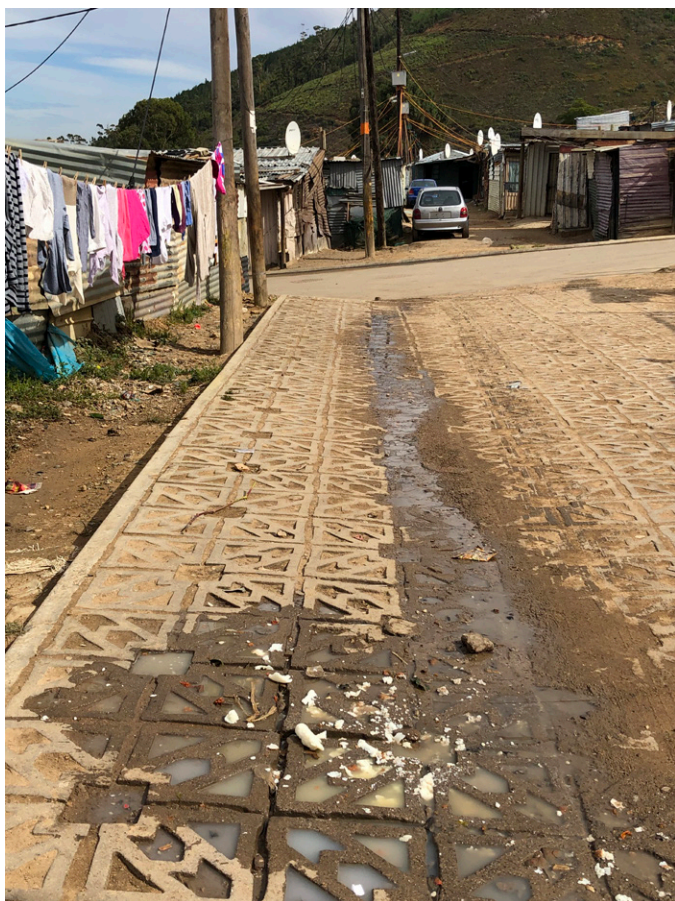
Constructed permeable paving between Block S and T.
