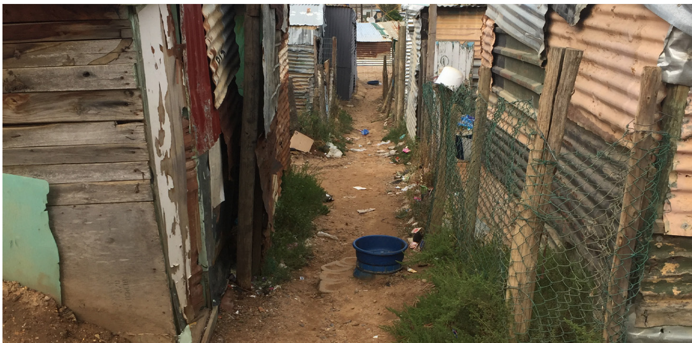
Installed greywater disposal point (blue drum).
